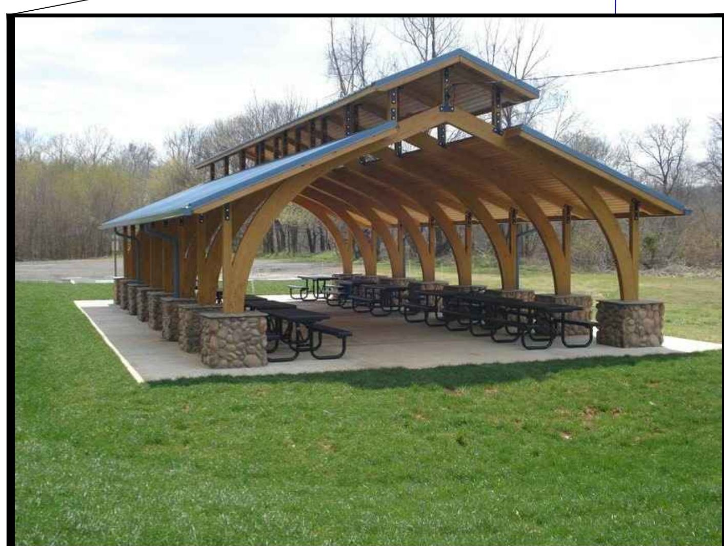
Common Area Structure
