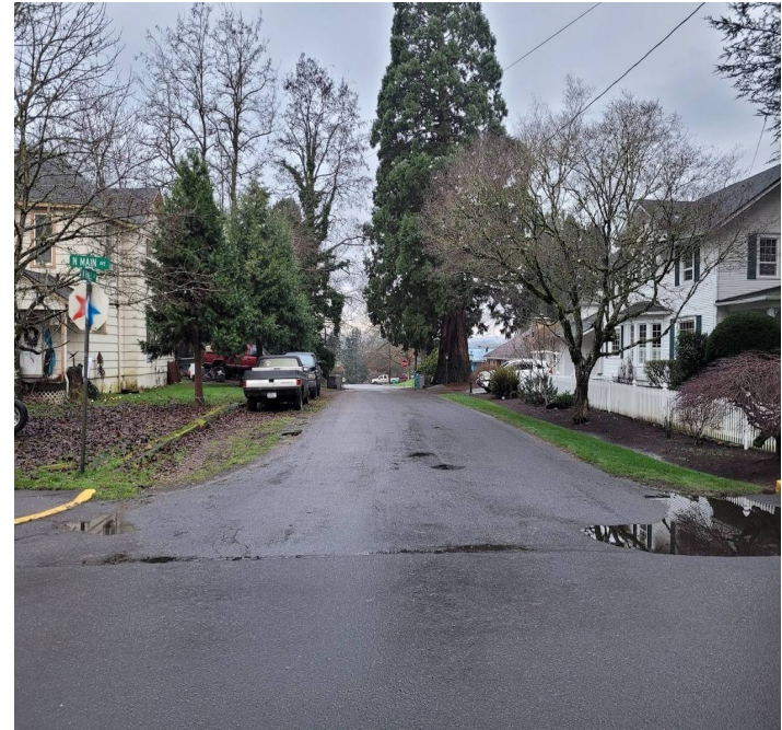
Curb, Sidewalk and Landscaping
