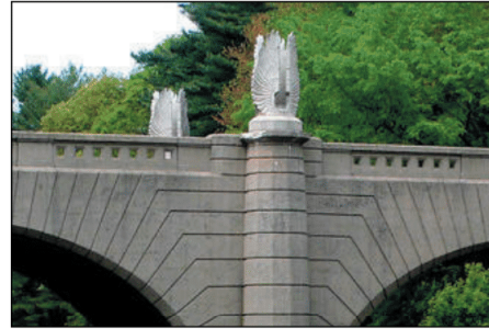
WPA Bridge with Noble Wings
