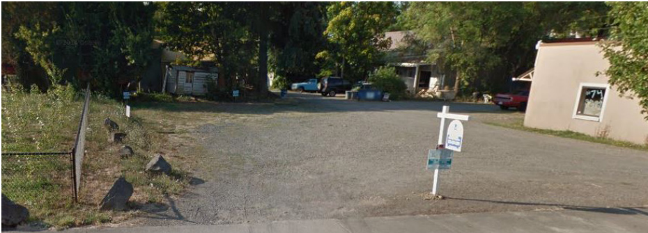
The Weeks Property is the gravel area on the right with the former gas station to the left.
