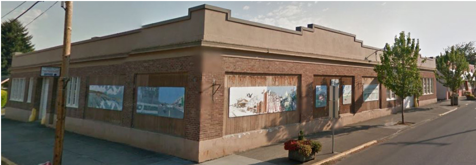
The Bus Barn at the corner of North 3rd Avenue and Pioneer Street.
