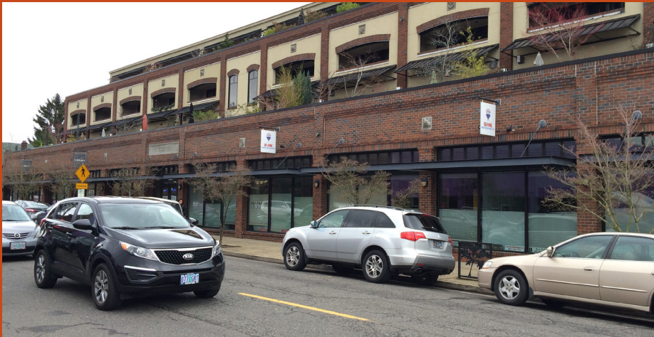
Multnomah County Library in Portland, Oregon is a three-story building, with each story recessed, that shares the ground floor with a realtor's office and supports apartments in the upper stories.
