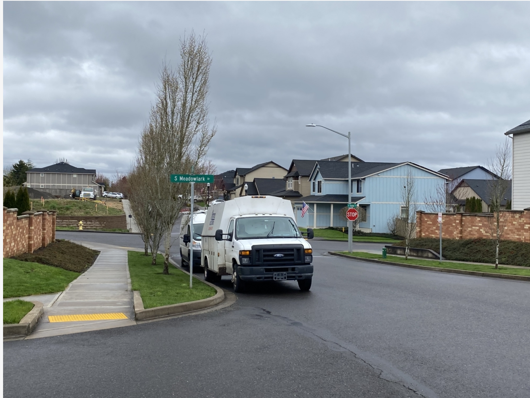
Parked vehicles impair sight distance turning from Meadowlark Drive onto Cispus Way toward Sevier
