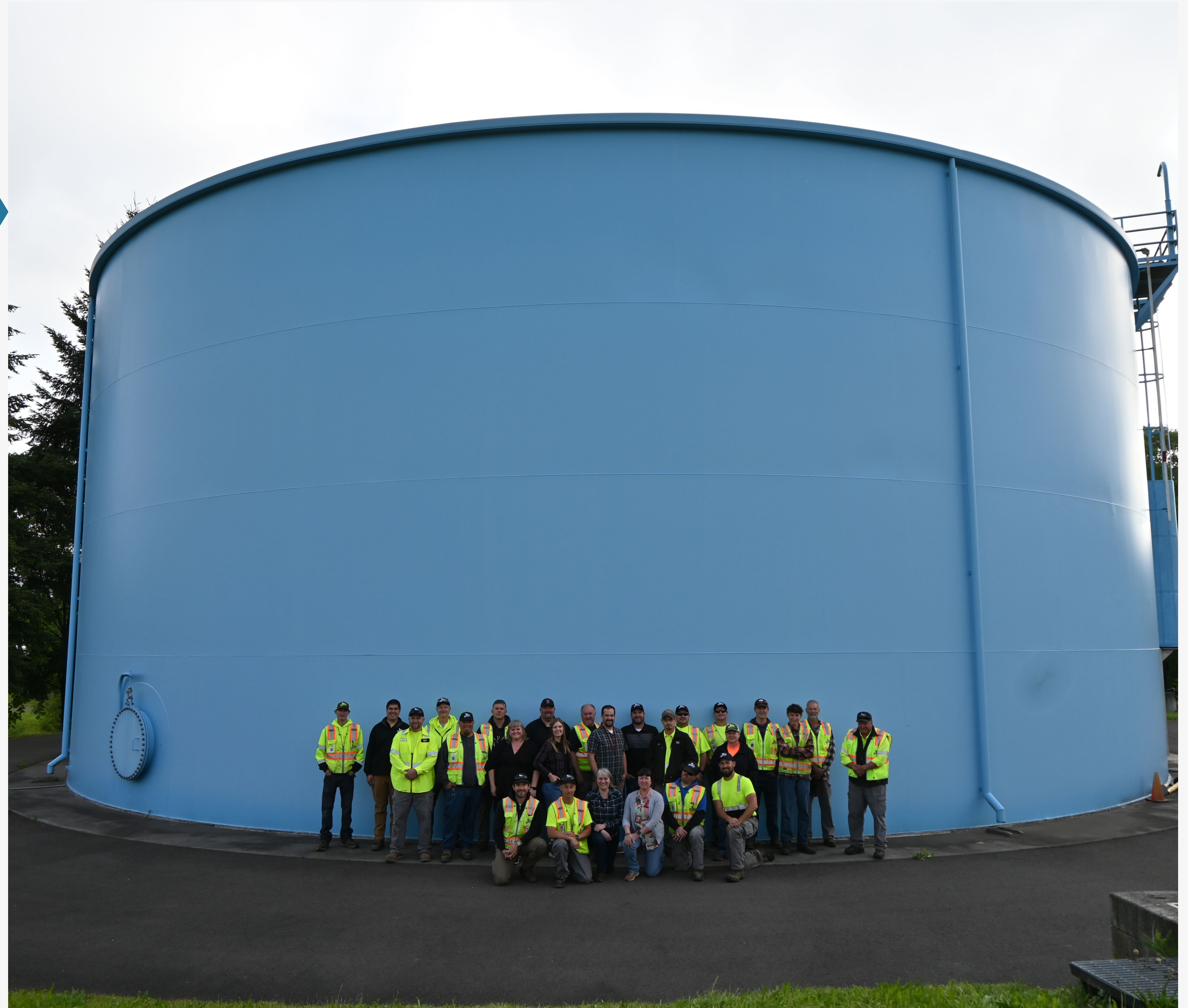
Junction one-million-gallon reservoir $1.98 million. Completed in 2017.
