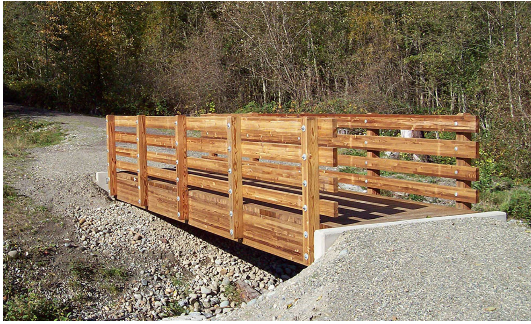
Pedestrian bridge at creek crossing
