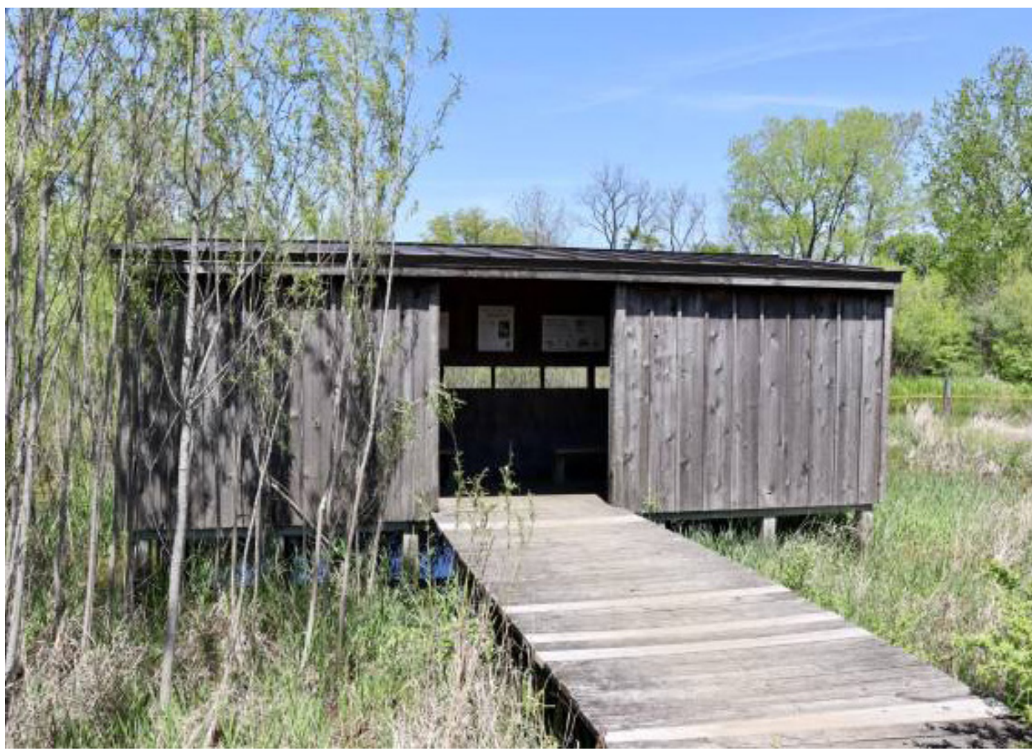
Wildlife viewing structures- bird blinds
