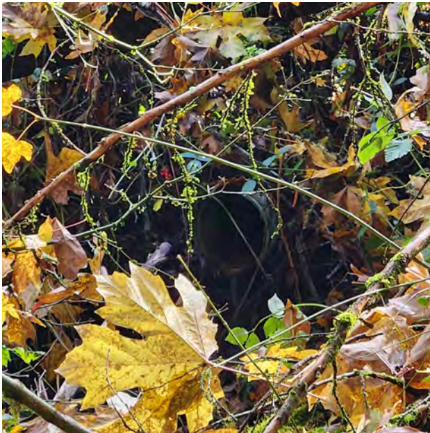
Photo 25. Culvert outfall from upper deepwater habitat (facing east).
