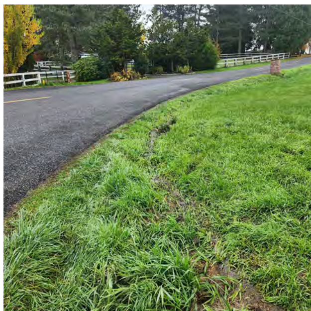
Photo 1. Wetland south of S 10 th Way (facing east).
