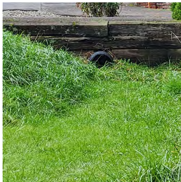
Photo 4. Wetland B outfall (facing west).
