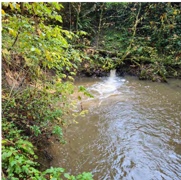
Photo 33. Culvert on other side of large logging road berm (facing east).
