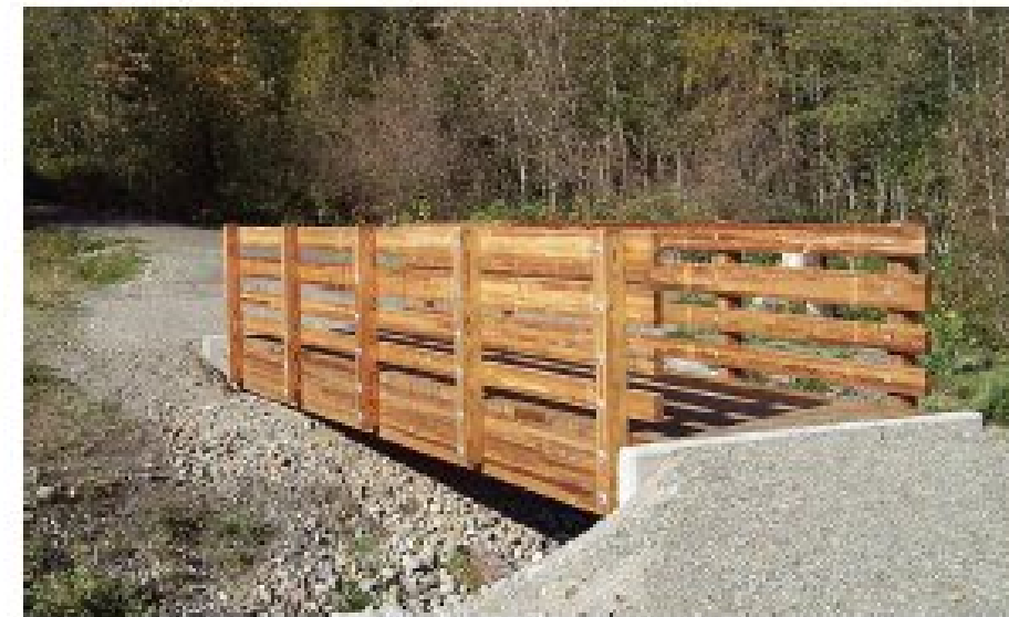
Pedestrian bridge at creek crossing
