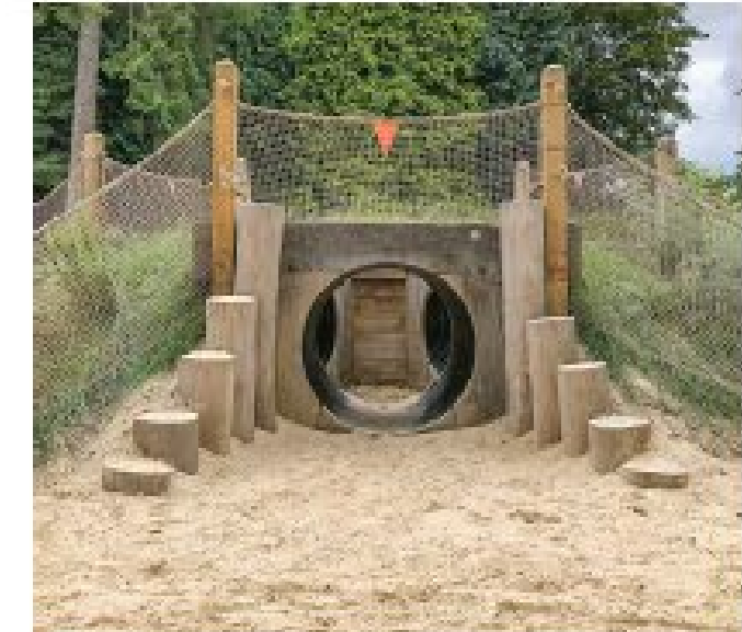
6 Tunnel through slope
