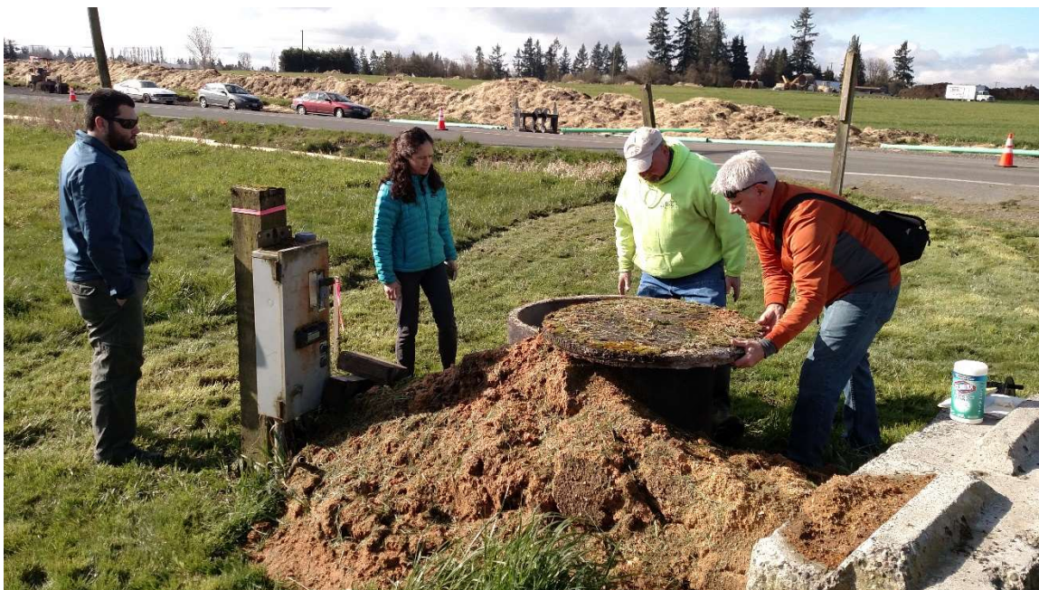
Photograph 6 – Well BAR-862 wellhead.
