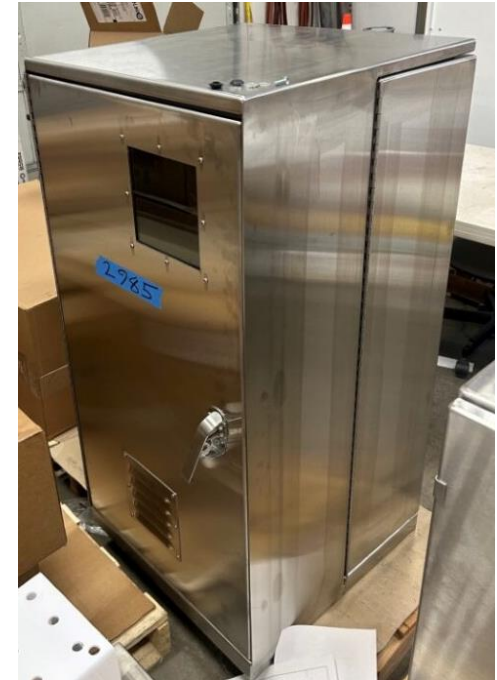
RTU Side Cell Antenna Window
