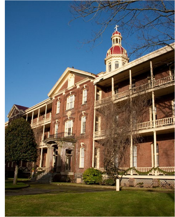
House of Providence, Built 1873
